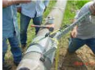
Step 3 - Tighten the Sleeve
