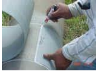
Step 2 - Mark and Apply the Sleeve
