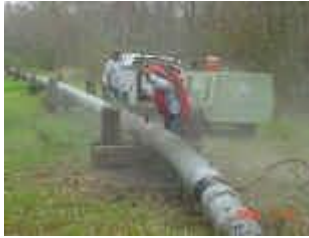
Step 1 - Prepare the Pipe Surface
