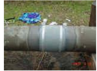
Step 4 - Completed Installation
