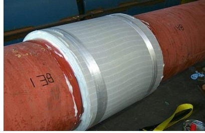
Completed Installation in 35 minutes
