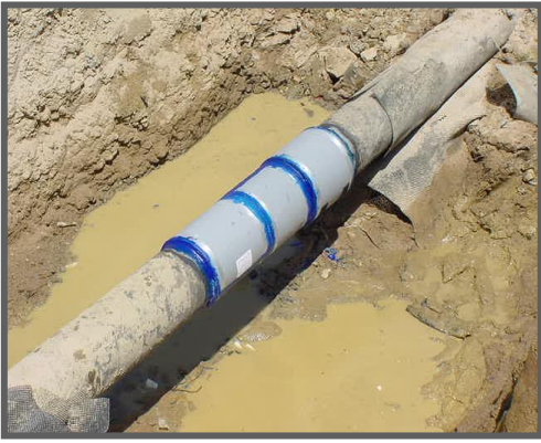
View of Several Sleeves “Butted” together
