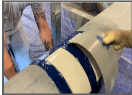
Securing the WeldWrap™ to Anchor Pad
