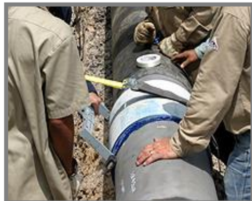
Positioning the Adjustable Torque Bar
